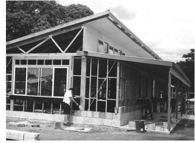
Community Childcare Cooperative building in progress
