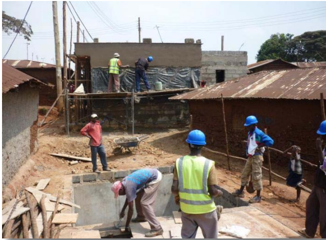
Figure 2: Construction of WASH facilities in Kibera slum, Nairobi, supported by WSUP
