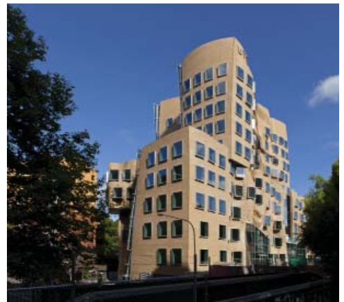
Exterior, eastern façade. Credit: Andrew Worssam
