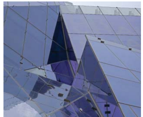
Glass 'curtain wall'. Credit: Andrew Worssam
