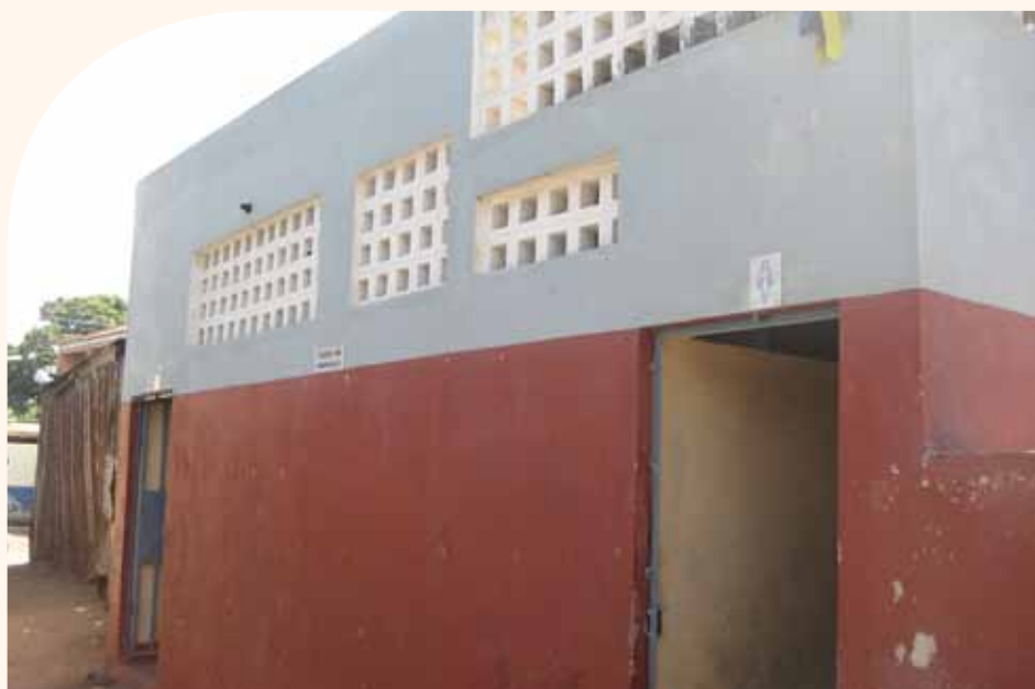
CARE/WSUP: Project sites in informal settlements in Maputo. Toilet block with facilities for women and men.
