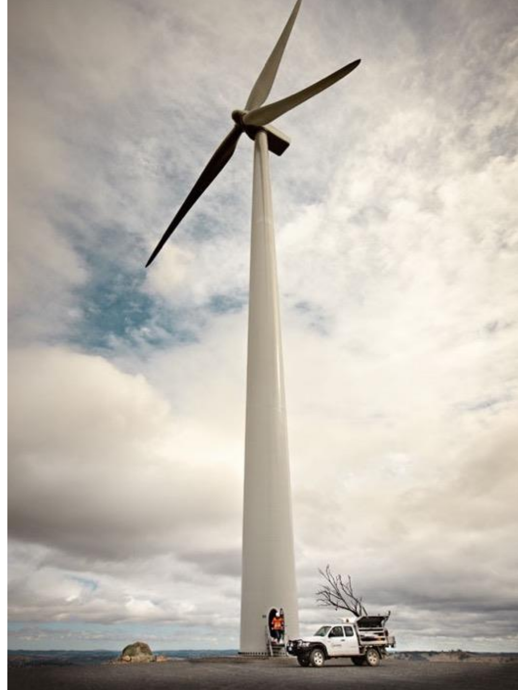
Photograph courtesy of ACCIONA Energy
