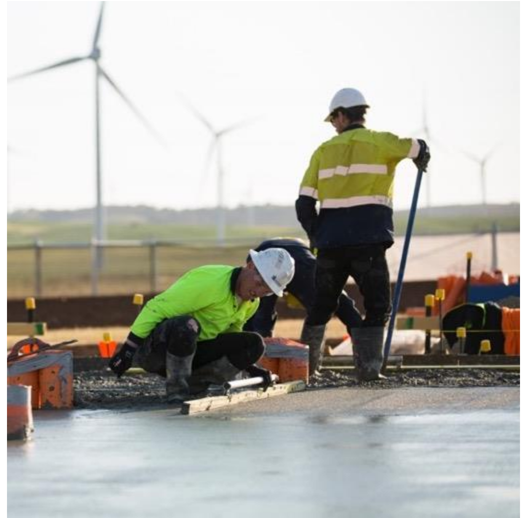
Photograph courtesy of Neoen
