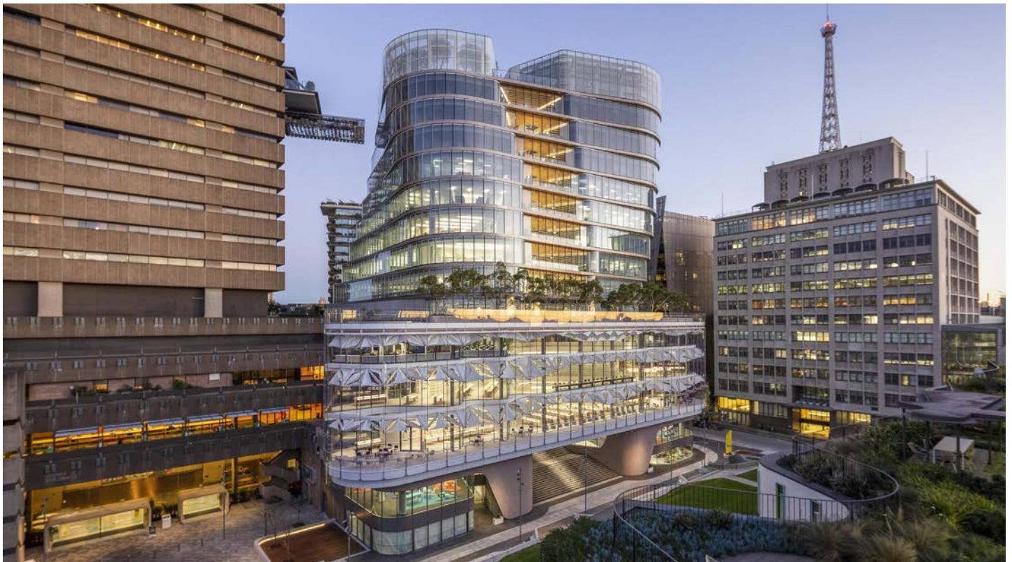
UTS Central, Building 2
