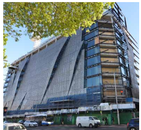
FEIT Building in progress. Credit: UTS
