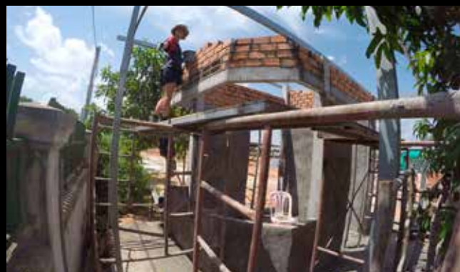
Constructing for Developing Communities in Cambodia. Photo: Michael Er
