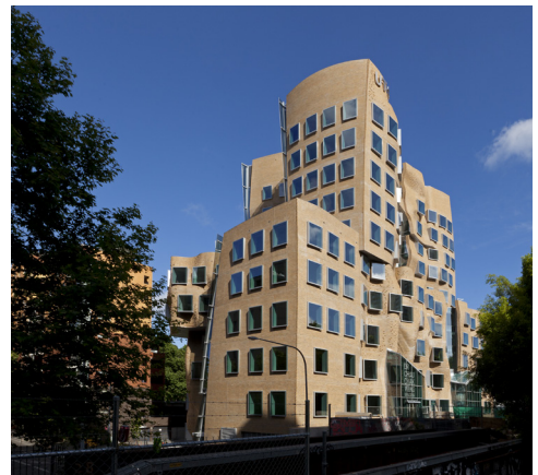
Exterior, eastern façade. Credit: Andrew Worssam
