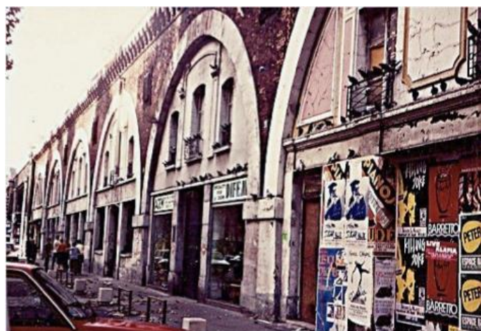
Figure 13. The viaduct de Bastille prior to the restoration. Source:
