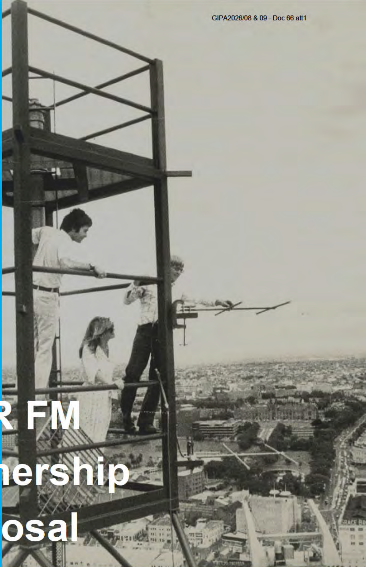
2SER antenna installation atop the UTS Tower Building, 1979
